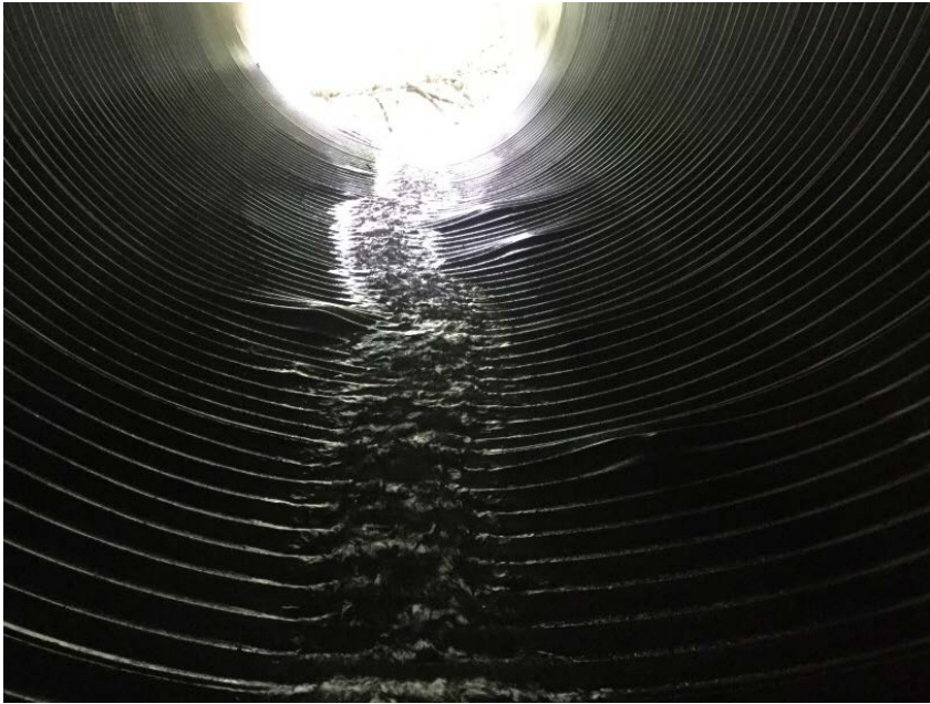
Minor damage to floor
